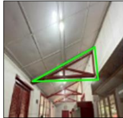
Figure 9. Roof Support Structure of the Museum
