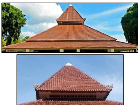
Figure 2. The roof of the main building
